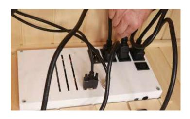
Plug in all heater leads to receptacles in the power supply box.
