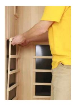
Reinstall the side wall heater guards
