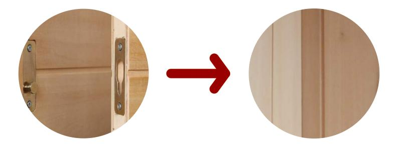
There are two sets of fasteners to join the saunas' back corners together. After lowering the Back Wall, check to ensure that both sets of fasteners have connected by looking at the corner inside of the sauna. It is possible to connect one set of fasteners and miss the other. If there is an obvious gap in the corner between the two walls the fasteners have not connected and the raising and lowering procedure will need to be repeated.
