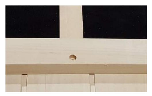
Screws are included to attach the heater guard to the wall. Select a drill bit with a smaller diameter than the screw threads to drill a pilot hole
