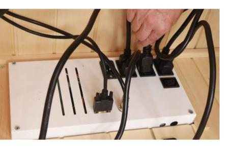
Plug in all heater leads to receptacles in the power supply box.
