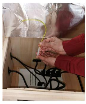
Connect the **grounding** wire from bottom side of Bench as shown
